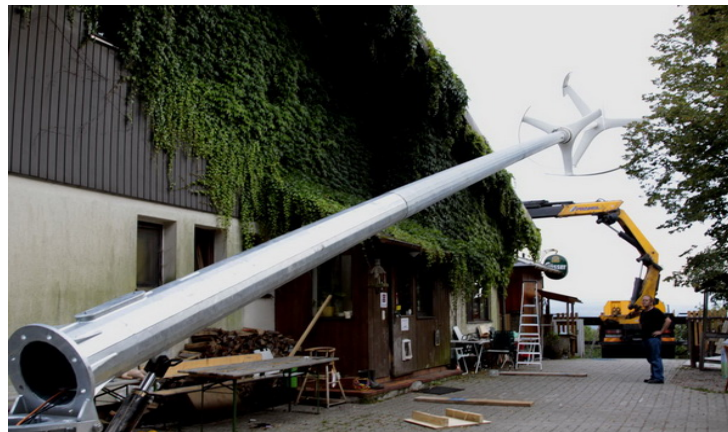
Figure 3 setting up the qr5 wind turbine
