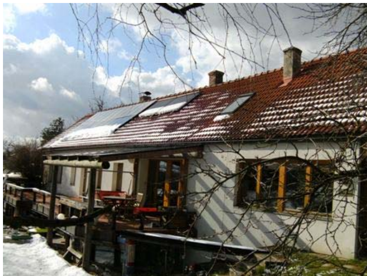
Figure 1: Building with photovoltaic & solar thermal
